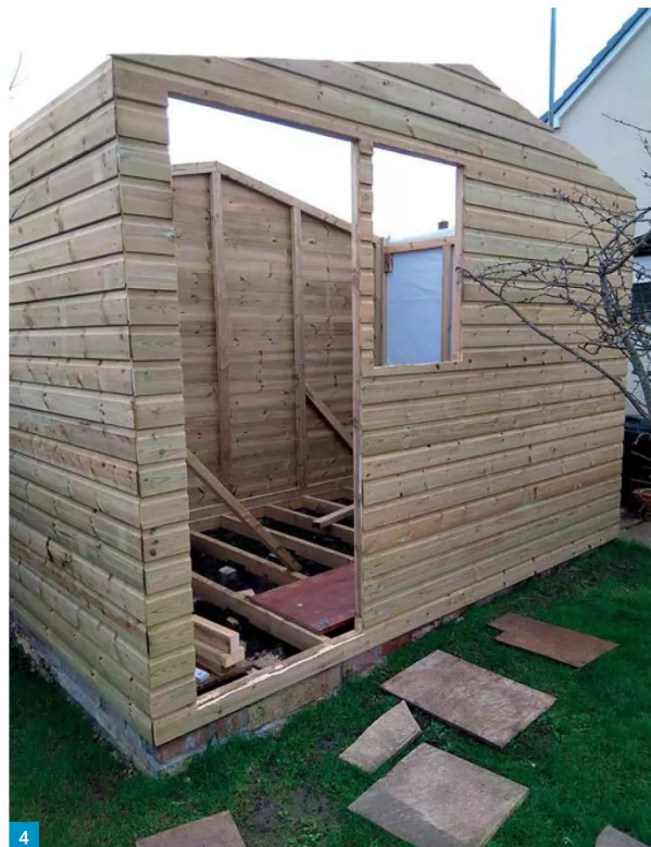
Fig. 1: Squeezing a base into the available space. Fig. 2: The rear was built horizontally ... Fig. 3: ... and then braced in its final position. Fig. 4: The completed cladding with gaps for door and window. Fig. 5: Composite beam for roof support.
